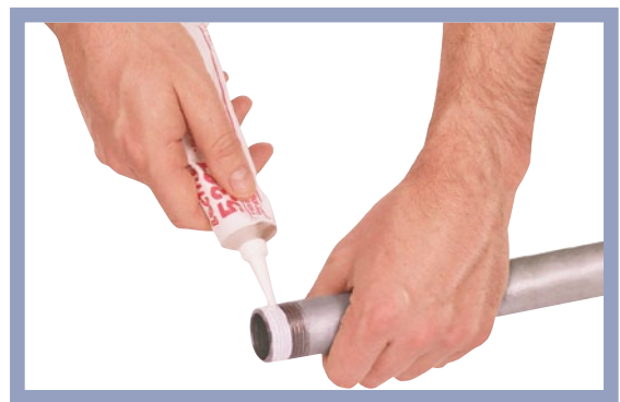
1 (b) thread paste sealant. The right sealant for threaded joints is non-hardening, compatible with plastic and doesn't add slipperiness to encourage over-torquing.
